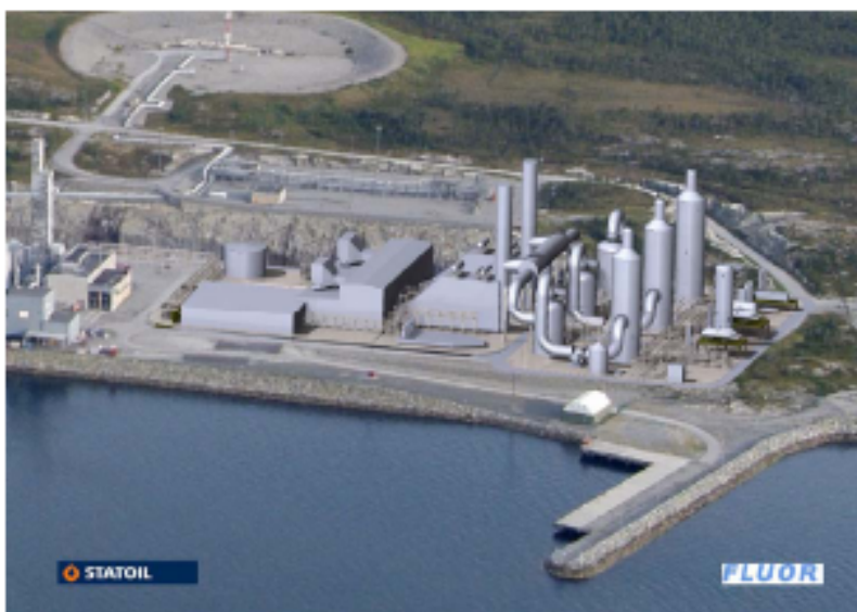
Figure 15: Tjeldbergodden: The planned CO 2 capture plant, to the right of the planned power plant (StatoilHydro and Fluor 2005)
